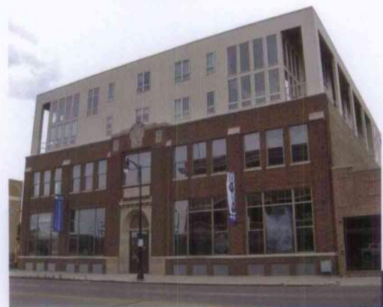
Figure 20. The height, as well as the design, of these two-story rooftop additions overwhelms the two-story and the one-story, low-rise historic buildings.
