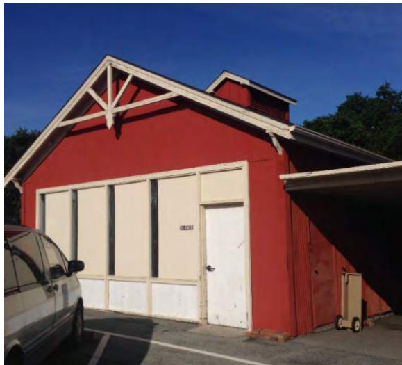
South Shed with corrugated metal siding. Source: UA/CPD March 2015.
