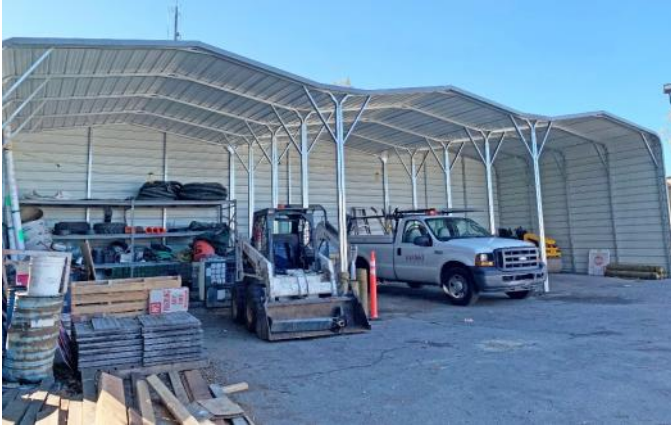
Figure 1: Three-bay steel-frame shed added ca. 2018.
