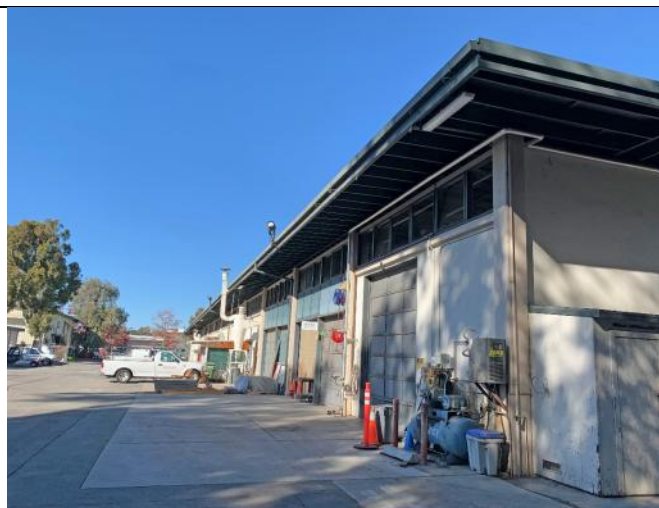
Figure 3: Looking northwest along southwest façade.
