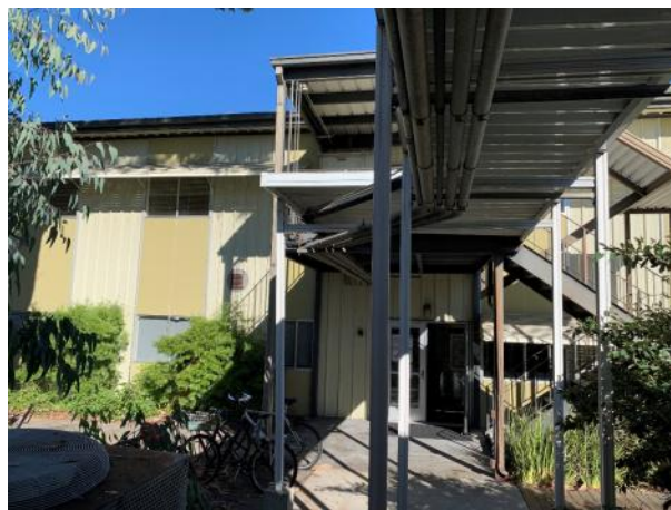
Figure 3: Southwest façade, looking northeast.
