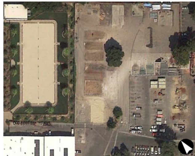
Figure 19: Aerial photo showing former northernmost section of Bonair Siding Corporation Yard cleared for redevelopment, September 1, 2017. Source: Google Earth.
