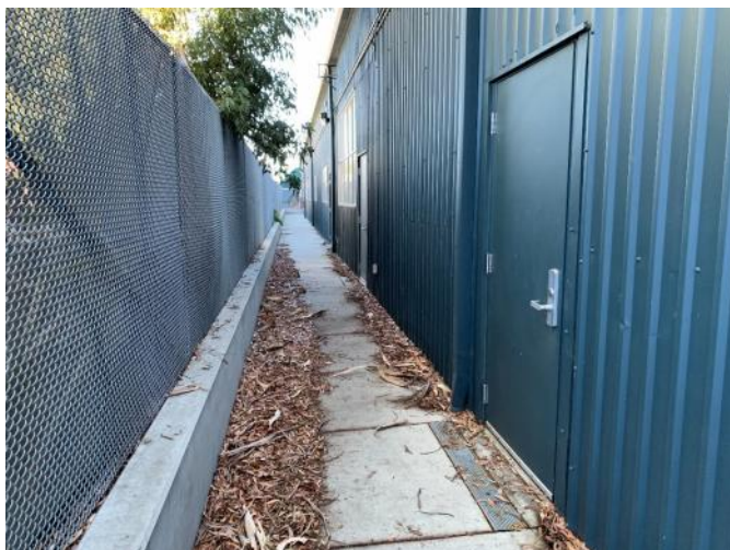
Figure 12: Fence separating rear façade from athletic facilities to the west, looking northwest.
