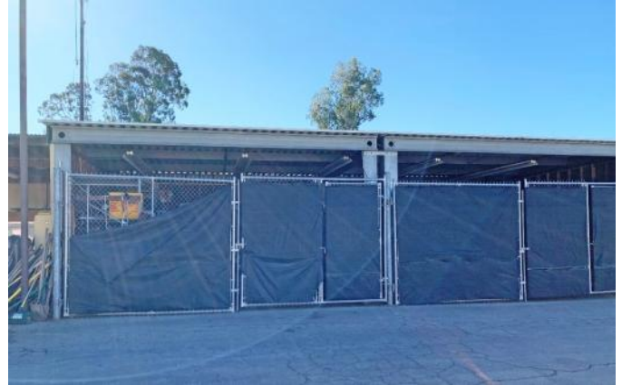
Figure 2: Steel-frame shed that was built in 1992.
