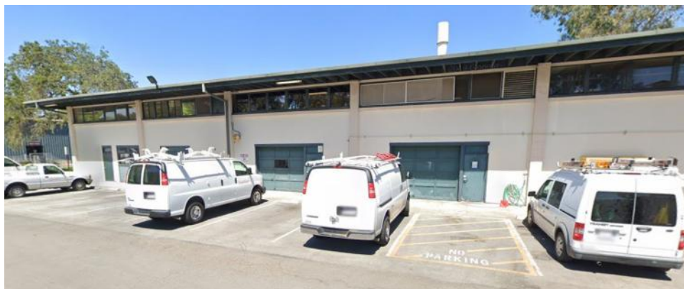
Figure 4: Rear southwest façade, looking north. Source: Google Street View, May 2019.
