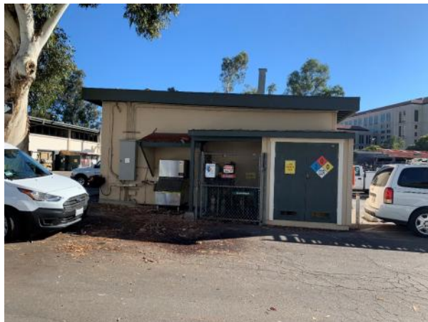
Figure 4: Northwest façade, looking southwest.
