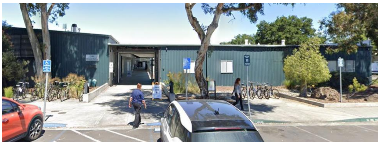
Figure 14: East half of the southwest façade, looking northeast.
