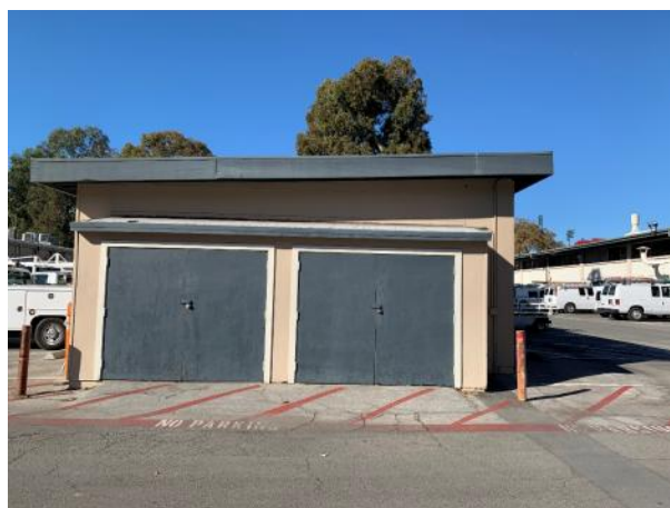
Figure 3: Southeast façade, looking northwest.
