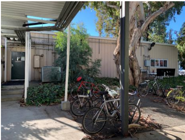
Figure 2: West end of northeast façade, looking southwest.
