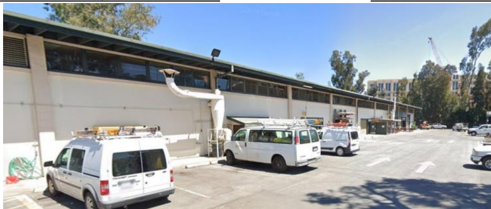
Figure 5: Rear southwest façade, looking east. Source: Google Street View, May 2019.
