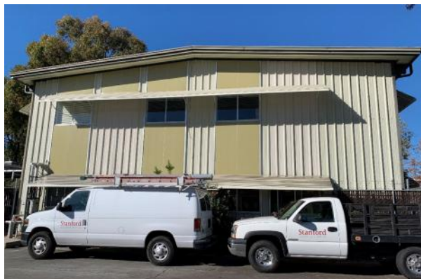
Figure 4: Southeast façade, looking northwest.
