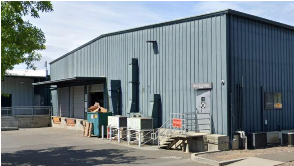
Figure 6: Looking north toward the 1987 stores warehouse addition. Source: Google Street View, May 2019.
