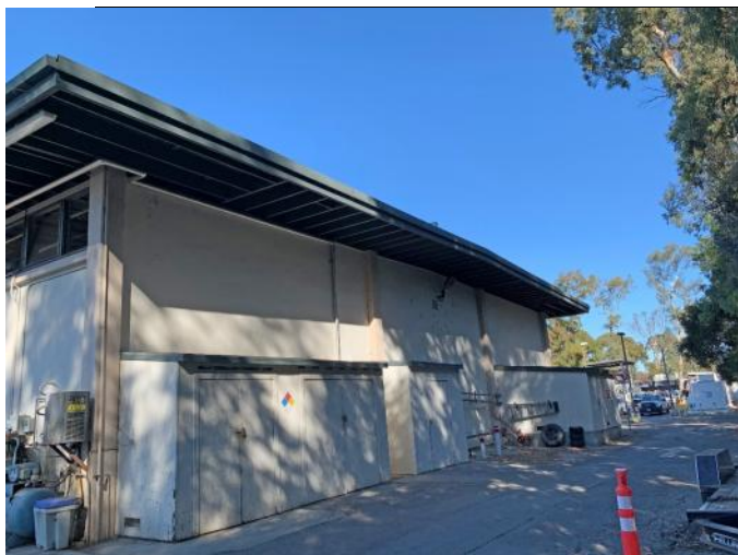
Figure 2: Southeast façade, looking north.
