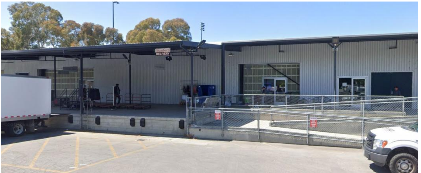
Figure 5: View of north half of the north half of the original section of the building, with loading dock, ramps, and altered garage bays, looking west. Source: Google Street View, May 2019.
