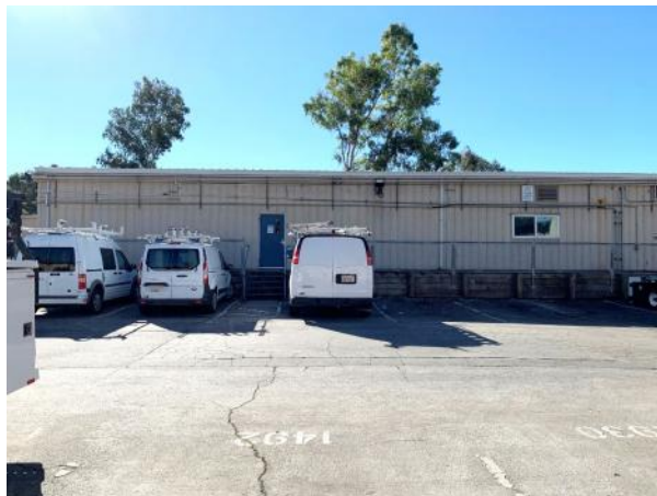
Figure 4: Rear portion of northeast façade, looking southwest.
