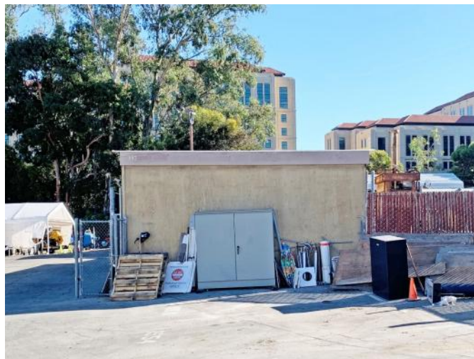
Figure 3: View of west side of 1992 steel-frame shed.
