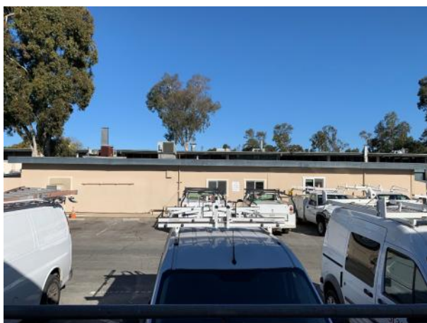
Figure 2: Southwest facade, looking northeast.
