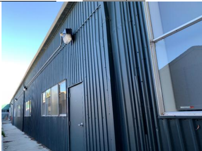
Figure 10: North end of rear façade, looking northeast.
