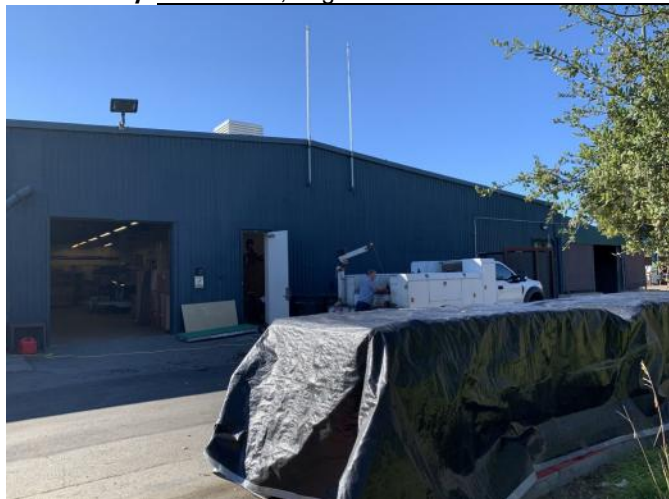
Figure 9: Northeast façade, looking west.
