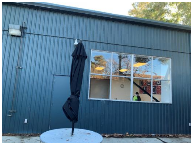
Figure 11: Steel-sash window in rear façade, looking northeast.
