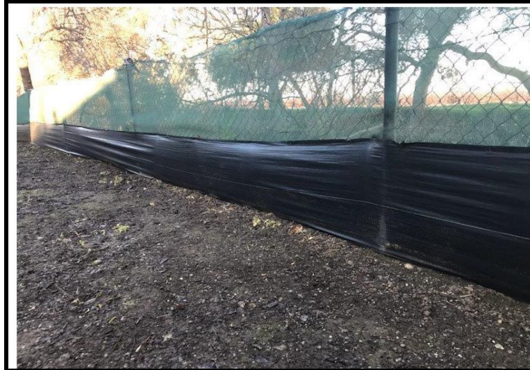
Figure–8 – Silt fence located north of the Christopher Ranch property line
