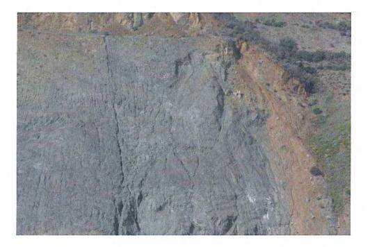
Photo 18: Wedge failure in the lower part of the western face.
