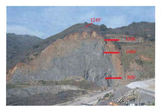
Photo 8: The west face. Note the change in color marking the irregular boundary between weathered and unweathered greenstone. The slope on the right is side cast fill. The elevations are approximate.
