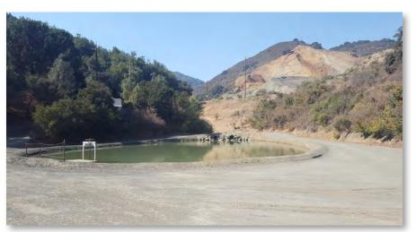
RPW-3, Third settling pond looking northwest. Culverts drain RPW-2 into RPW-3 seasonally.
