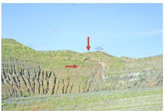
Photograph 2. The east end of the north face, looking north. The horizontal arrow marks the 2019 landslide. The vertical arrow marks pad 1. The white band marks are on the east quarry face and are a possible indication of water seepage.
