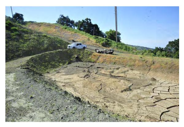
Photograph 5. The settling pond, looking NW. Water enters the pond through the pipe visible below the truck.
