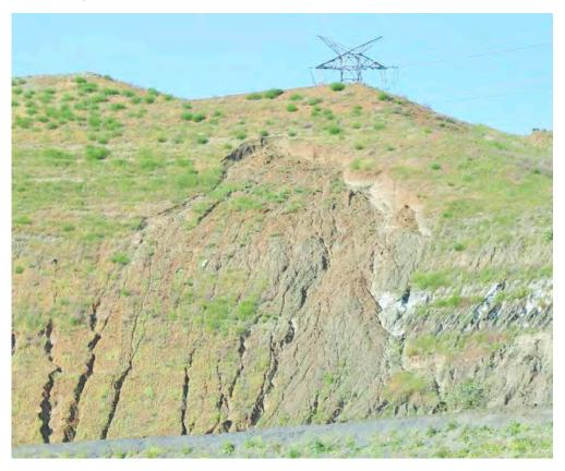
Photograph 3. An enlarged area from Photograph 2. The landslide is visible and Pad 1 is above the landslide. The landslide toe does not extend to the bottom of the slope.
