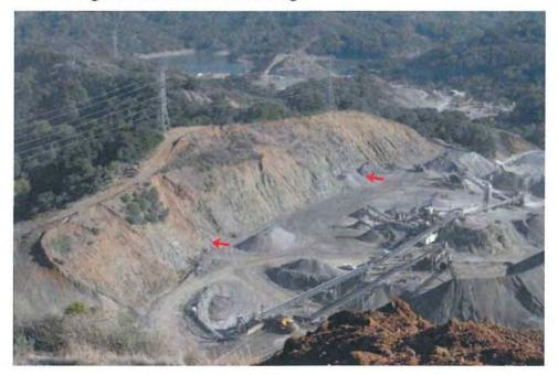
Photo 16: The east face (weathered greenstone). The arrows indicate landslides where machinery has removed the toe of the slope and caused landslides (see photograph 21). The Berrocal fault is semi-parallel to and just on the other (east) side of the power lines.
