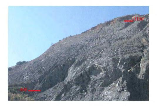
Photo 14: Wedge failures in the lower part of the western face.
