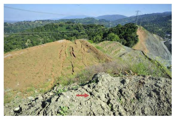
Photograph 8. Ground cracks at the south end of Pad 2 (visible in Photo 7). Looking from Pad 1 (foreground). The cracks extend into Pad 1 (arrow).
