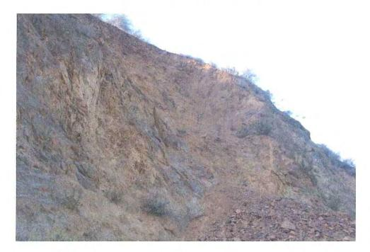
Photo 20: The failure in the middle of the upper bench. This is a progressive spalling failure rather than a wedge failure. Note the small size of the debris. This face is about 40 feet high. 21: A landslide in the
