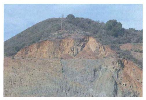
Photo 19: The upper bench in the west face. Note the localized failures. This face is more than 17 years old.
