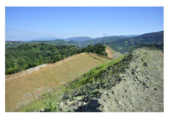
Photograph 7. Pad 2 as viewed from Pad 1. Ground cracks are visible at the south end of Pad 2.
