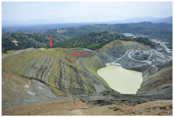
Photograph 1. An oblique view, looking east towards the NE corner of the quarry (from the NW corner). The horizontal arrow marks the 2019 landslide. The vertical arrow marks pad 1.
