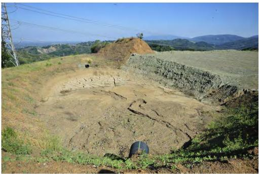
Photograph 4. The settling pond at the north end of Pad 1, looking east. Water flows into the pond through the pipe in the foreground. It leaves the pond through the pipe opening (black dot) in the far bank. Pad 1 is on the right. Note the bathtub rings that mark water levels in the pond.
