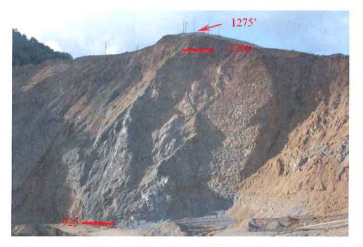
Photo 13: The north face. The reddish-brown slopes on either side of the center of the face are side-cast fills.
