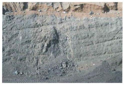
Photo 15: An apparent wedge failure in the shear zone in the northwest corner of the quarry. This is, instead, a spalling failure. A narrow zone along a vertical shear plane began to fail. There was then progressive spalling laterally away from the shear. The cliff at the wedge failure is about 40 feet high.
