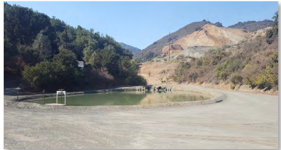
RPW-3, Third settling pond looking northwest. Culverts drain RPW-2 into RPW-3 seasonally.
