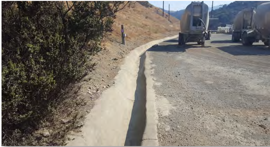
Non-RPW-1, Concrete lined ephemeral drainage looking southeast.
