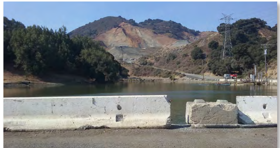
RPW-4, Fourth settling pond looking northwest from dam.
