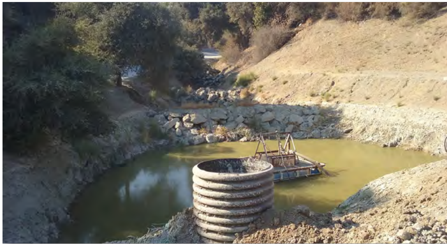
RPW-5, Small dammed basins cascading into settling pond, looking northwest.
