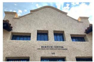
Figure 5: Shaped parapet, looking south.
