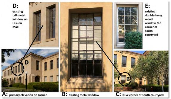
Figure 34 – Tall existing metal windows on primary façade (A, D). Metal and wood windows at north-east corner of southern courtyard (B, C, E) Source: UA/CPD
