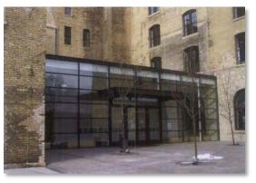
Figure 15 – "A glass and metal structure was constructed in the courtyard as a restaurant when this 1839 building was converted to a hotel. Although such an addition might not be appropriate in a more public location, it is compatible here in the courtyard of this historic building."<sup>39</sup>
