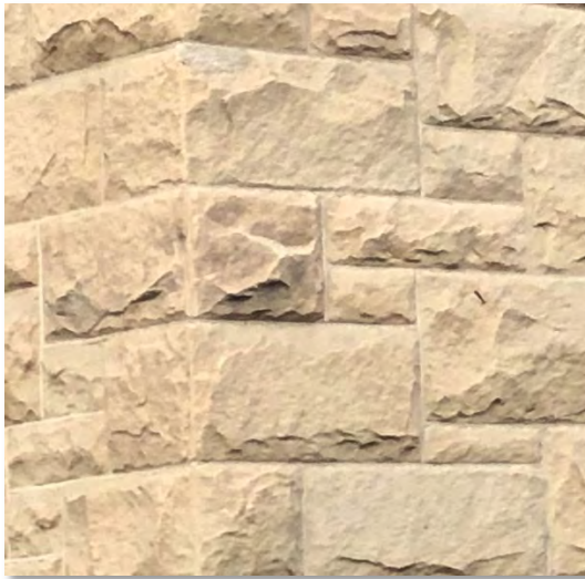
Figure 31 rusticated-chiseled typical sandstone with randomized jointing
