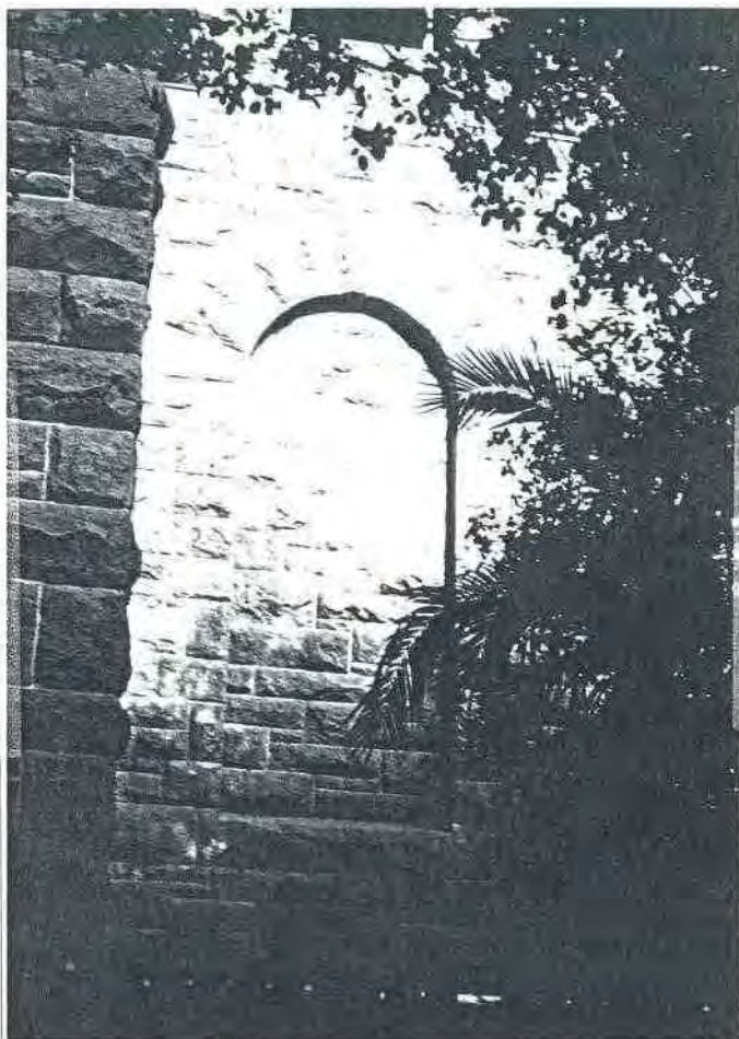
Photograph 2. Filled in window.
