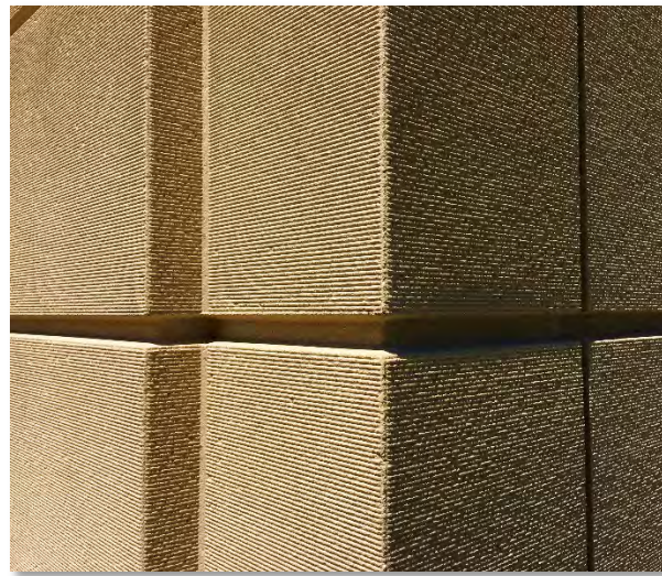
Figure 32 warm buff-tone precast envelope with fine and coarse aggregate finish with panelized jointing
