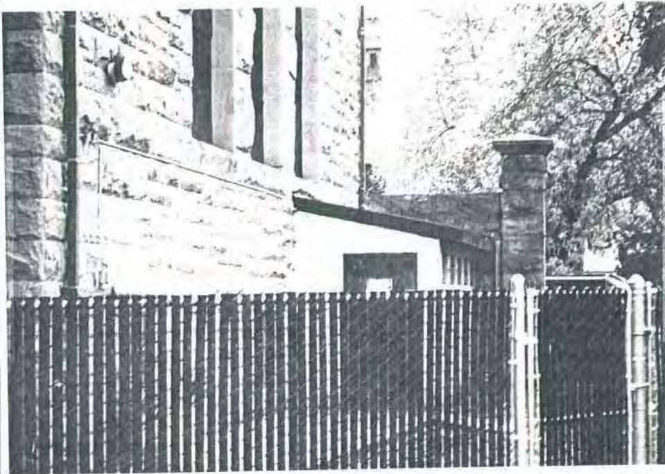
Photograph 5. Concrete block addition.
