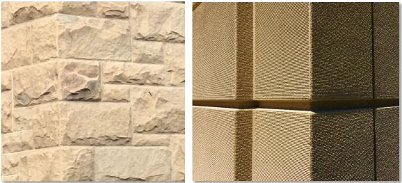
Figure 31 rusticated-chiseled typical sandstone with randomized jointing
