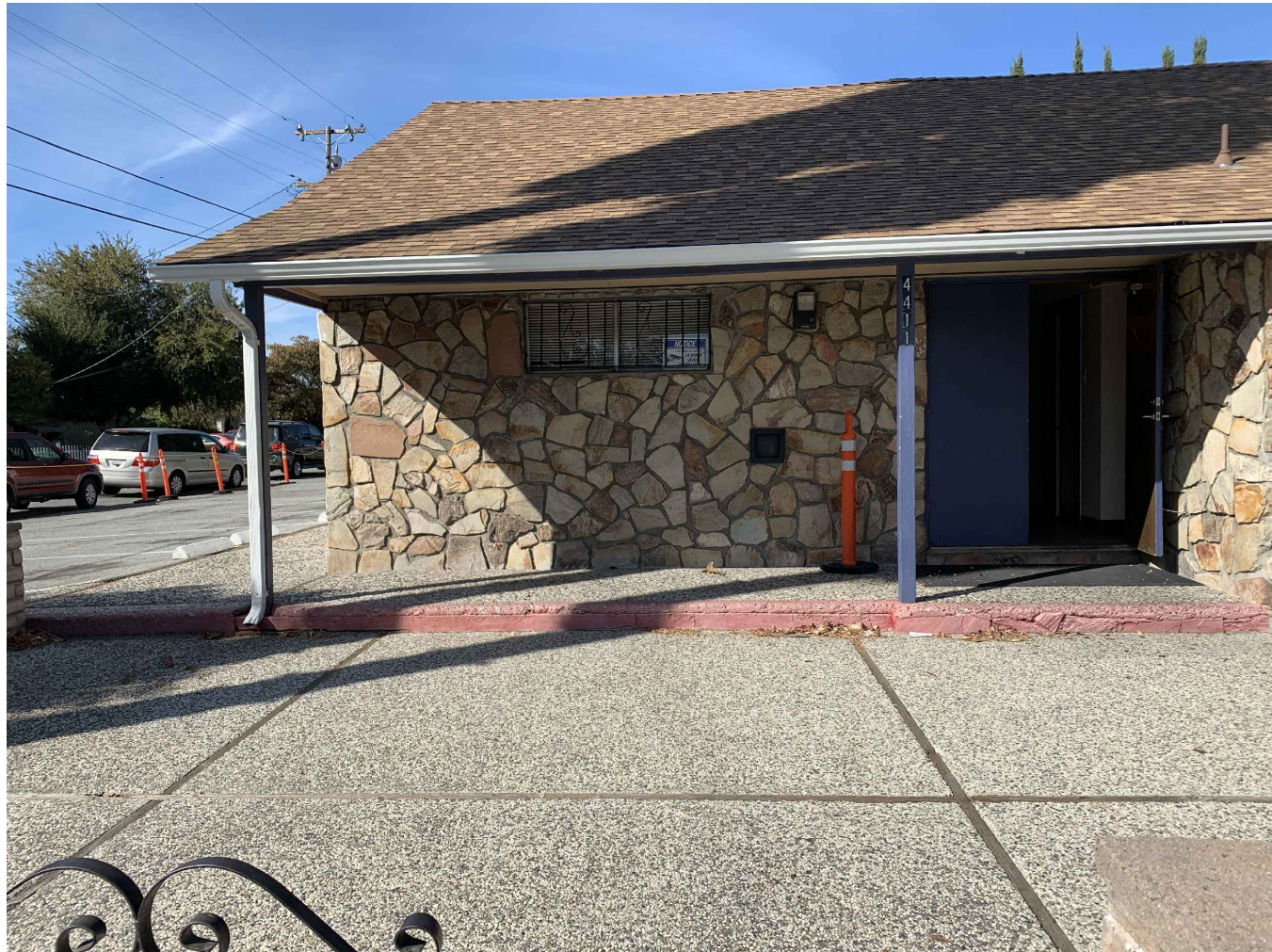
EXISTING STONE VENEER ON FRONT ELEVATION
