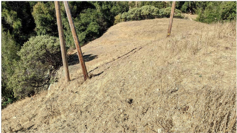
November 4, 2020 Slide Area Photos - As graded
