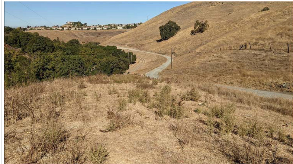
SLIDE AREA CONDITIONS AFTER FILL PLACEMENT
