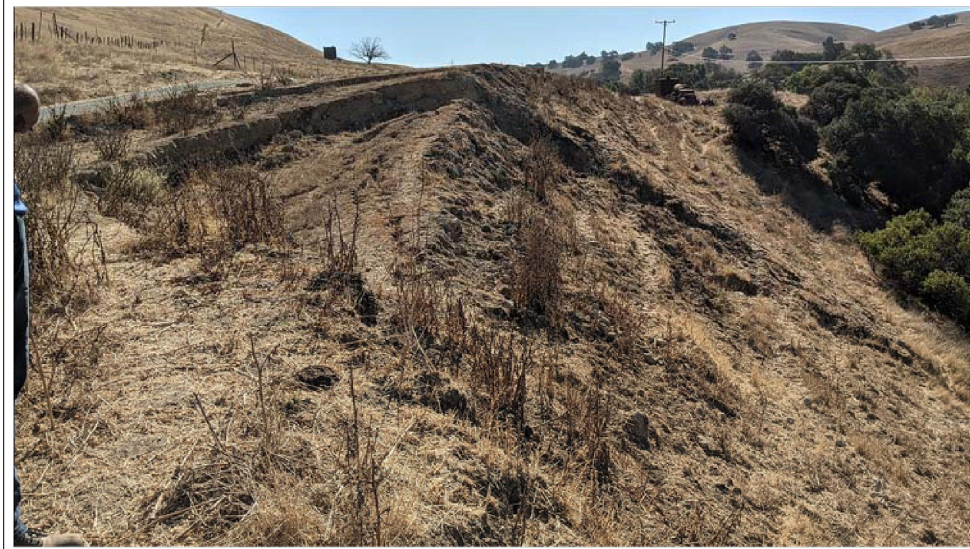
SLIDE AREA CONDITIONS BEFORE FILL PLACEMENT
