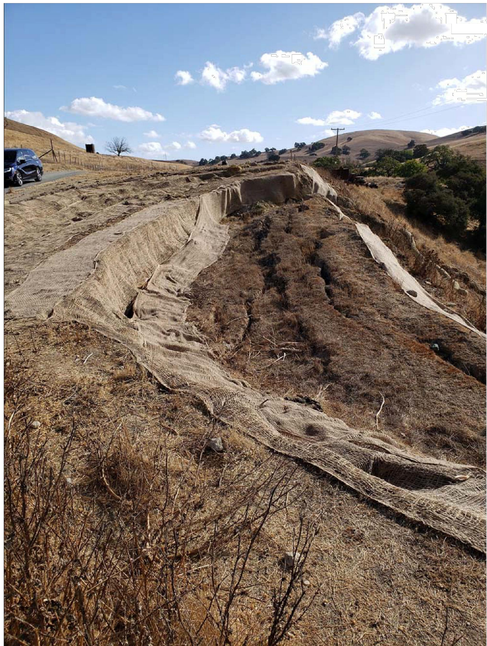
SLIDE AREA CONDITIONS AFTER FILL PLACEMENT
