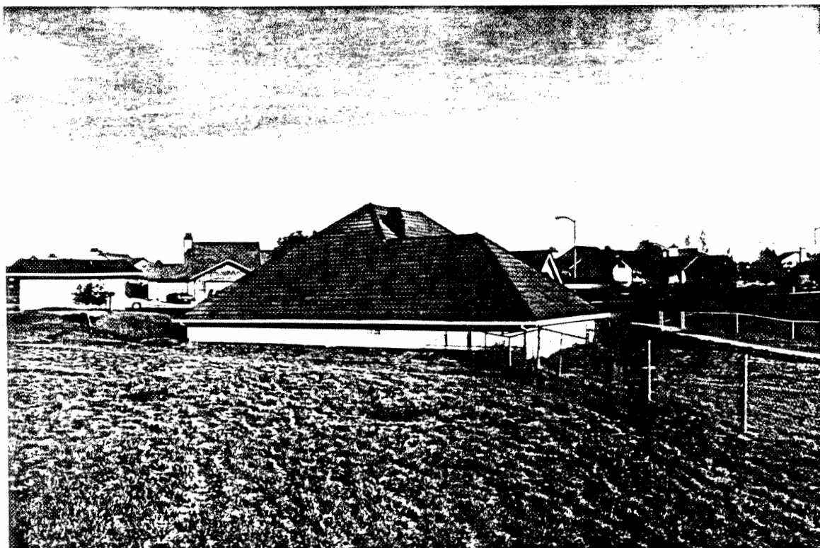
100,000 gallon per day facility in residential neighborhood, enclosed in house structure Fluidyne, Inc. SBR Equipment
