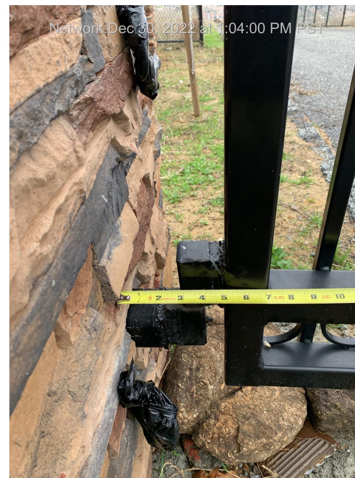
B: Gate Hinge-Column: 4" Gate Hinge-Hinge: 16'-11"
