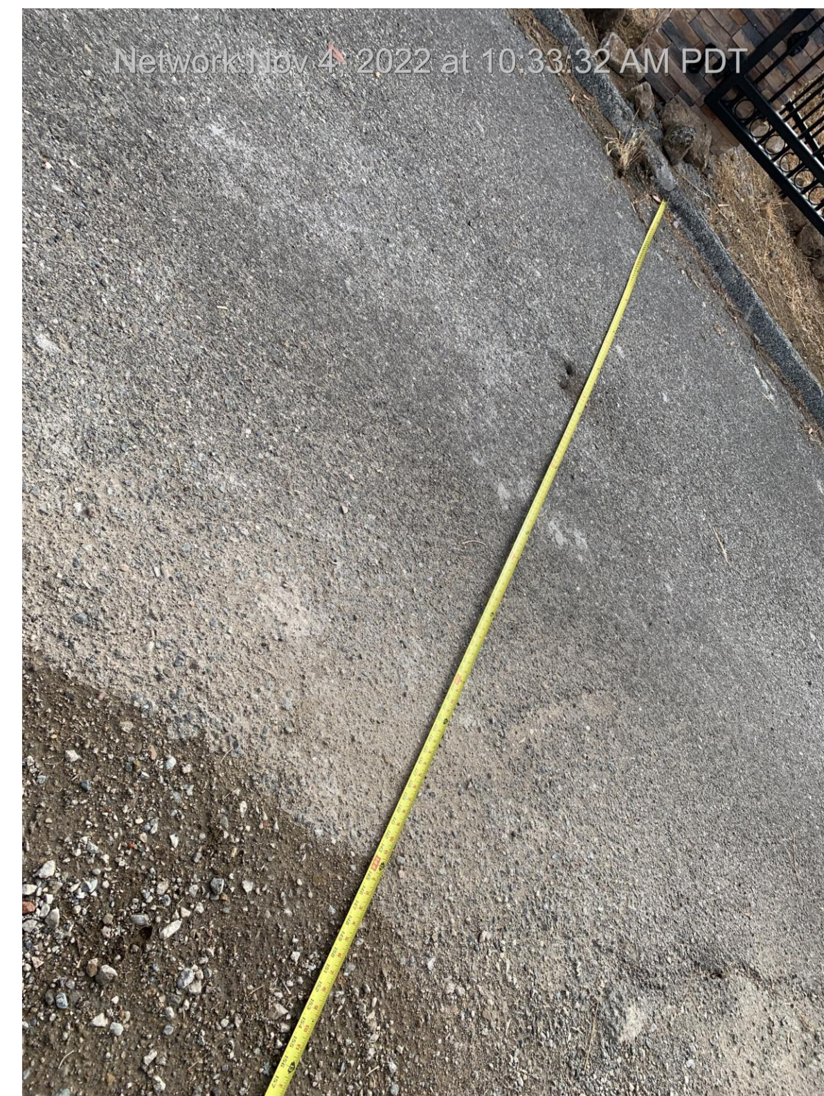
B: Driveway at Gate 12'
