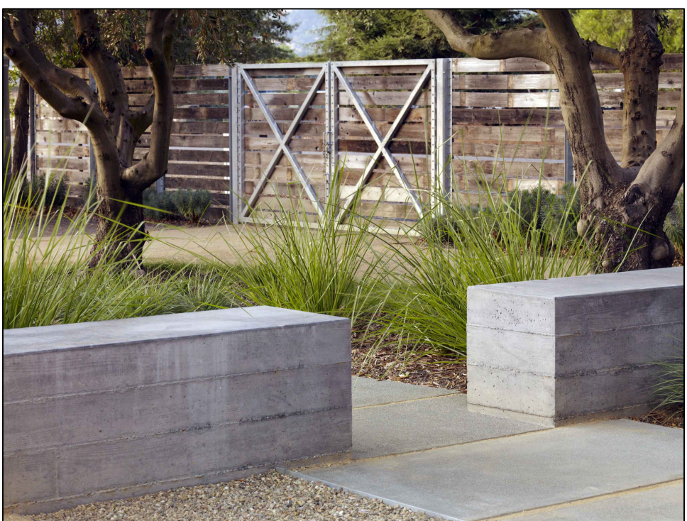
BOARDFORM CONCRETE WALL 3
