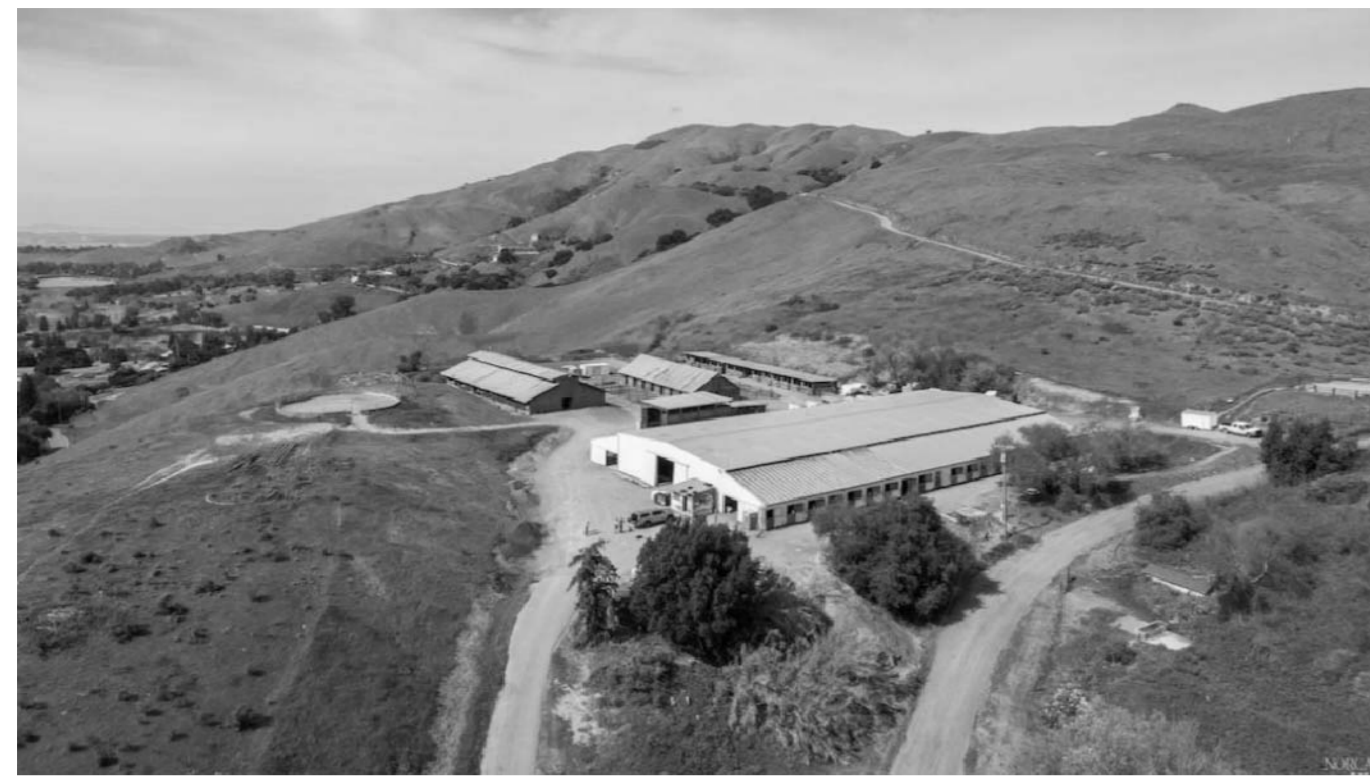
1. Previous Ranch (Demolished in 2019)
