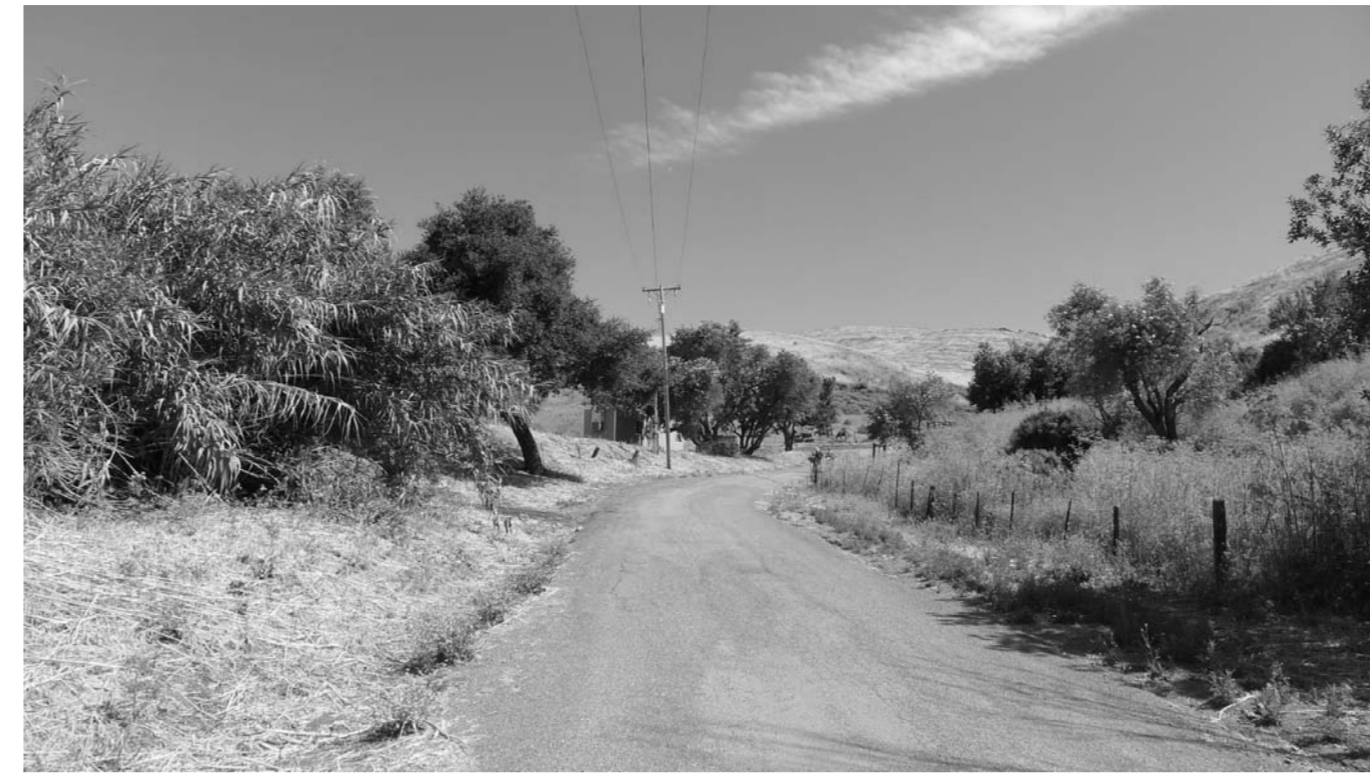
3. Weller Road Approach
