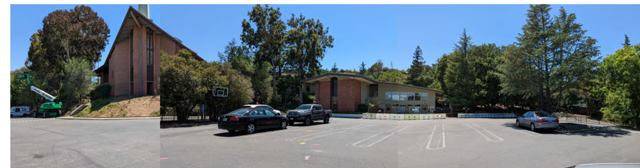
EXISTING VIEW AT LOWER PARKING LOT - NORTH
