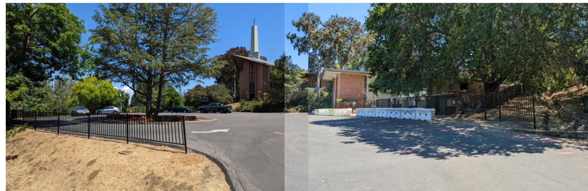
EXISTING VIEW AT LOWER PARKING LOT - EAST
