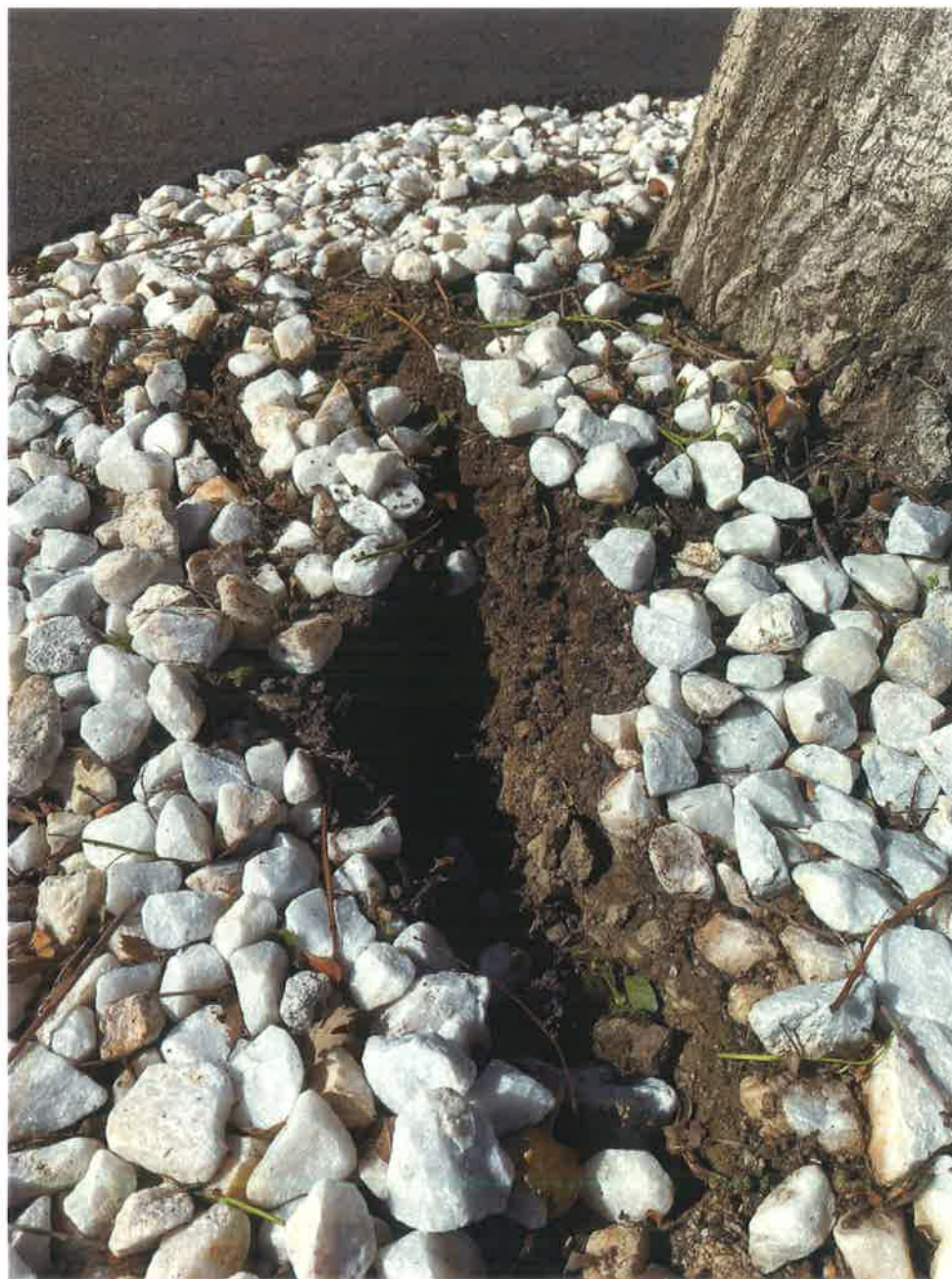
Photo 2. Soil separation and root destabilization were observed, the tree is leaning on other trees near by.
