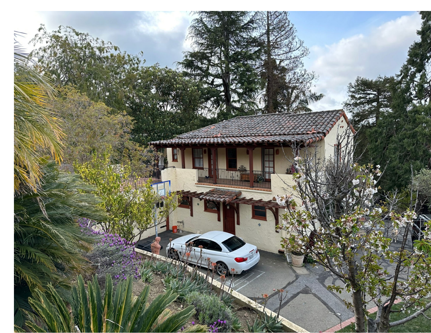
VIEW OF REAR FROM PATH UP
