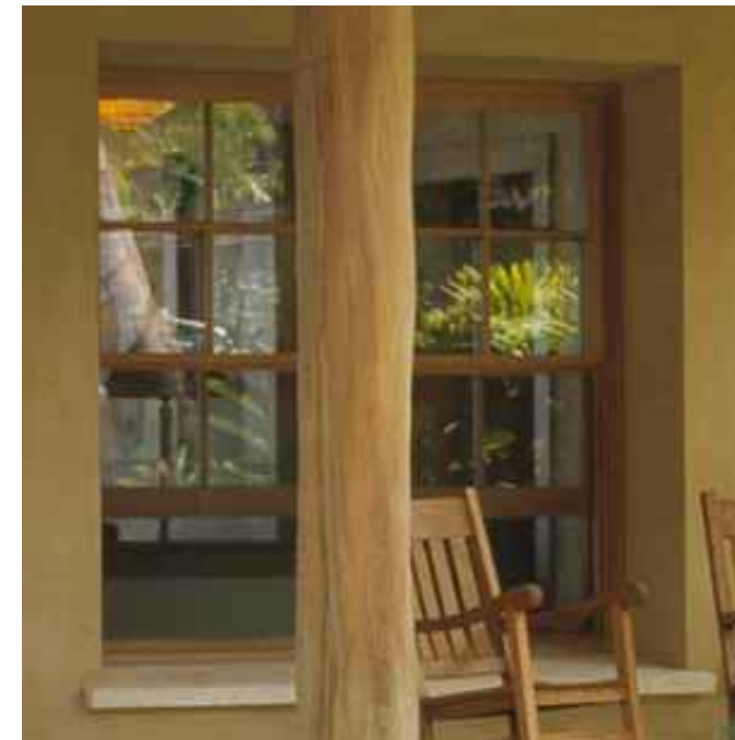
PROPOSED ALUMINUM FRAME WINDOWS AND DOORS BY MARVIN OR EQUIVALENT; RECESSED STUCCO WITH CAST/STONE SILL
