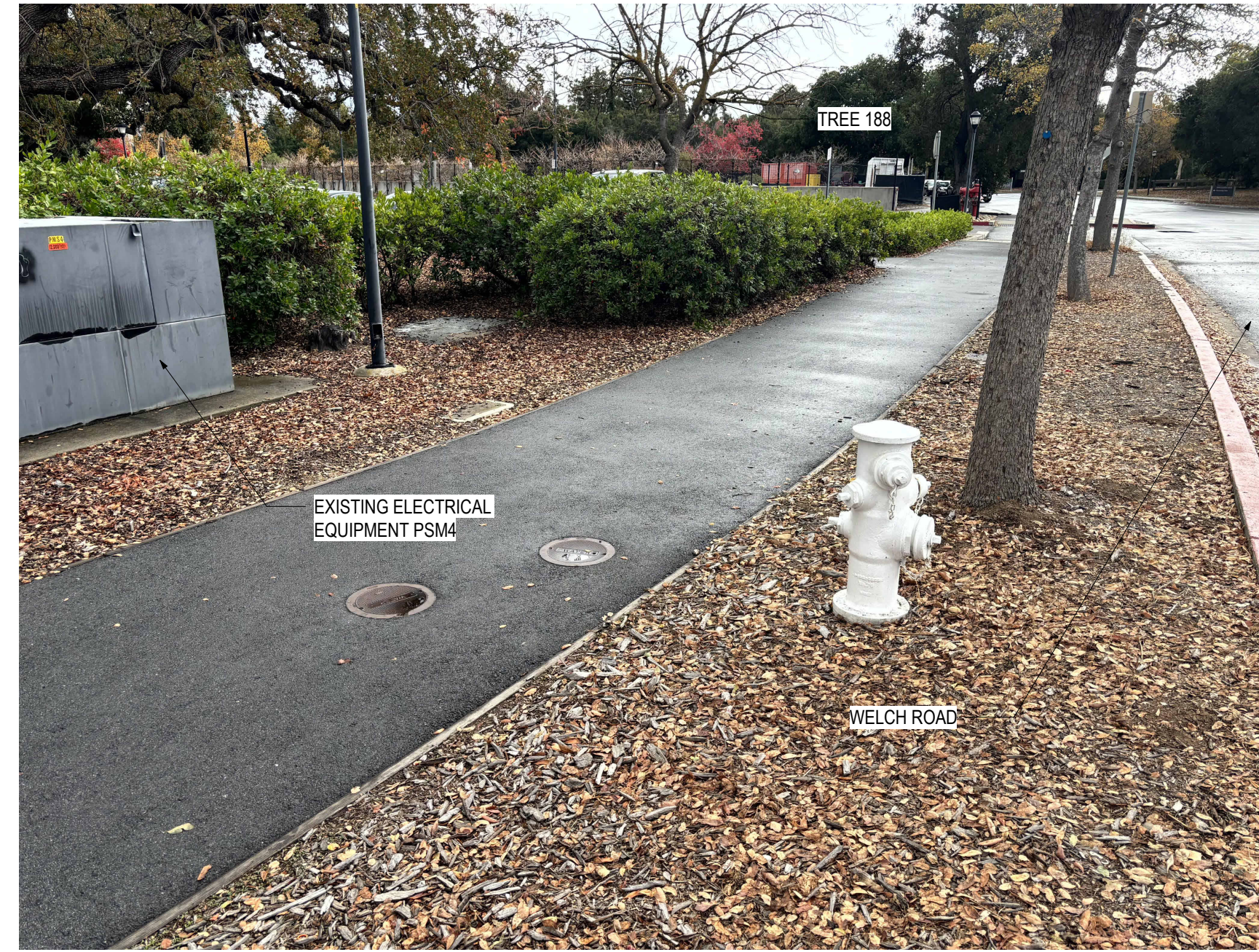
5 WELCH ROAD SIDEWALK AND UTILITIES
