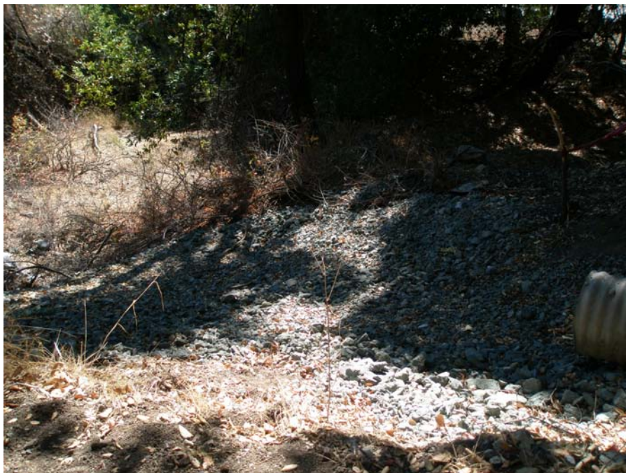
Photo 18: Pond 30 outfall to Permanente Creek, relined with greenstone. Dated September 26, 2013.
