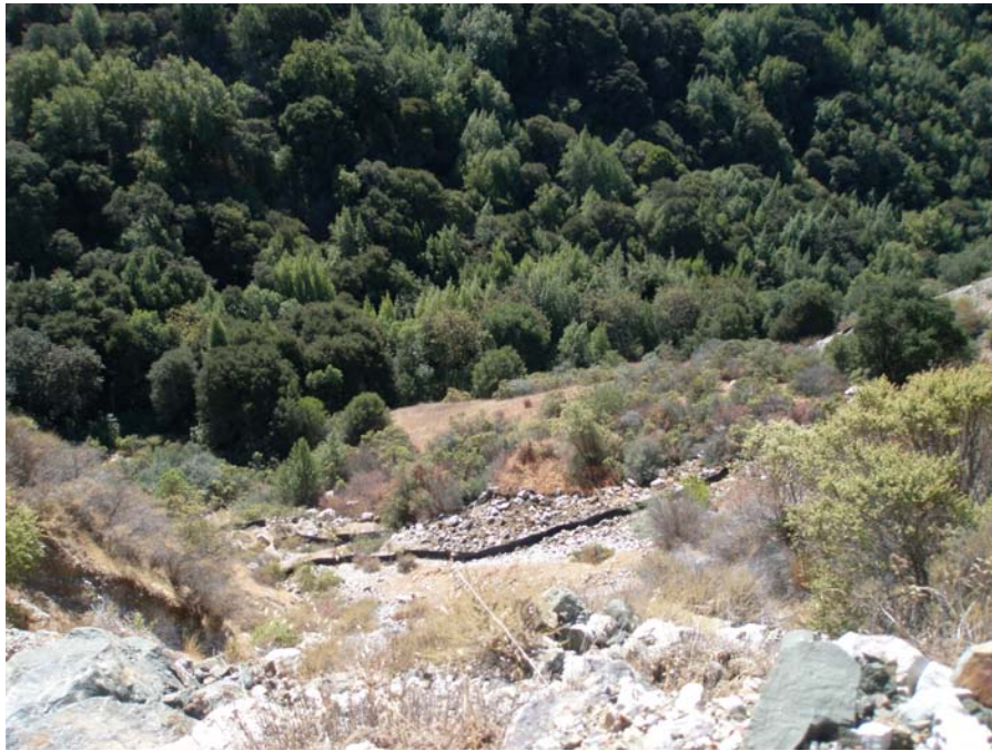
Photo 11: Silt fencing on southern slope of WMSA below outfall in Photo 9. Note soil mixed with talus adjacent to silt fence may be result of past slide. Dated September 26, 2013.
