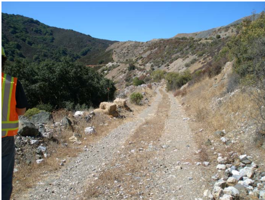
Photo 10: Straw waddles and bales at outfalls of mid-slope bench on southern slope of WMSA, looking looking west. Dated September 26, 2013.
