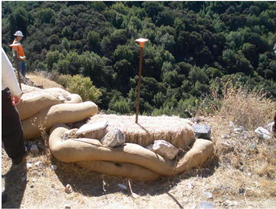
Photo 9: Rocked outfall in mid-slope bench on southern WMSA slope with straw waddles and bales, looking southwest into Permanente Creek. Dated September 26, 2013.
