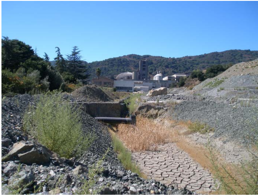
Photo 17: Pond 30 lowest pond in EMSA and drains into Permanente Creek, looking south at cement plant. Walls of pond and drainage ditch relined with greenstone. Dated September 26, 2013.
