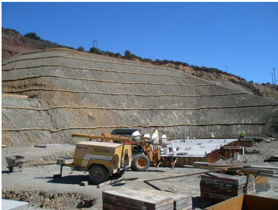
Photo 20: New secondary crusher pad area, looking northeast. Note straw waddles on slope. Slope will be hydroseeded before this winter. Dated September 26, 2013.
