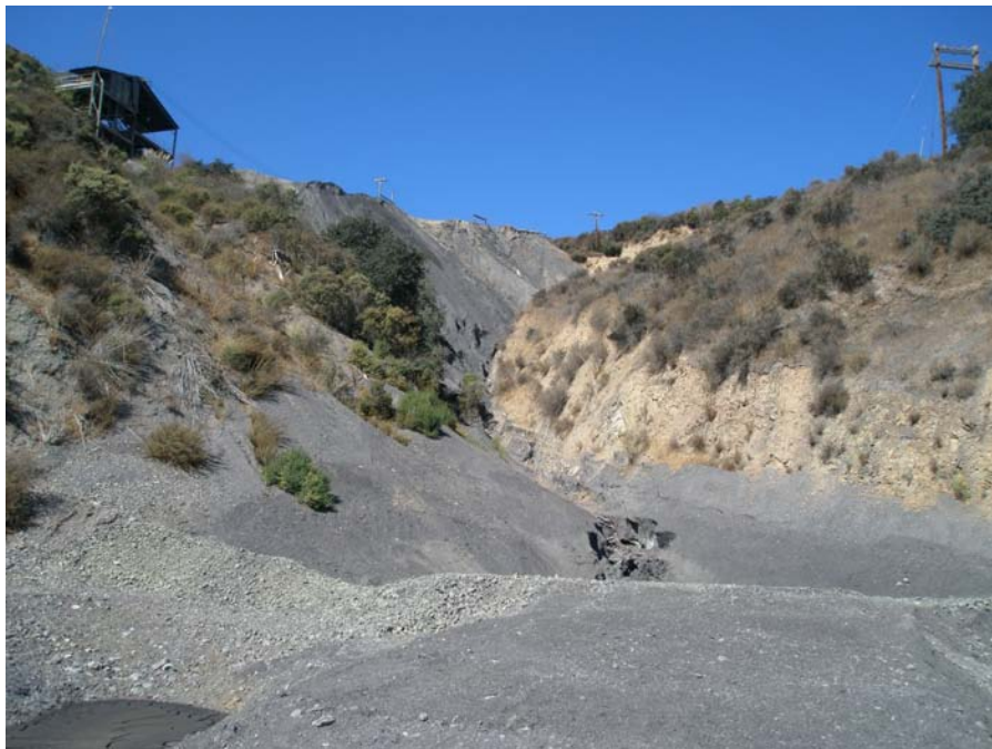
Photo 14: Slope failure north of eastern end of 500-foot long conveyor tunnel in Crusher/Support Area, looking west. Sediment catch basins constructed above western perimeter drainage ditch in foreground. Dated September 26, 2013.
