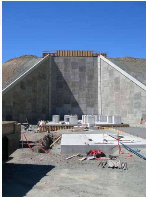
Photo 19: New primary crusher structure, looking west. Drainage from area will be collected and pumped into North Quarry for treatment before discharge. Dated September 26, 2013.
