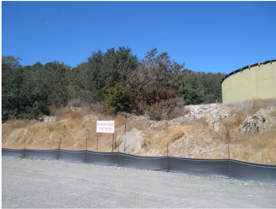
Photo 13: Topsoil storage area EMSA with sign and silt fence, looking west. Abandoned water tank at right side of image. Dated September 26, 2013.
