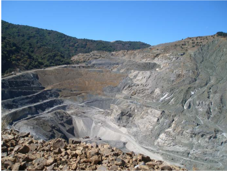
Photo 1: North Quarry, southwest portion. Waste rock material being placed at toe of western slope. Potential “Haul Road Slide” in eastern slope of WMSA, right of image. Floor elevation of quarry at approximately 725 feet msl. Dated September 26, 2013.
