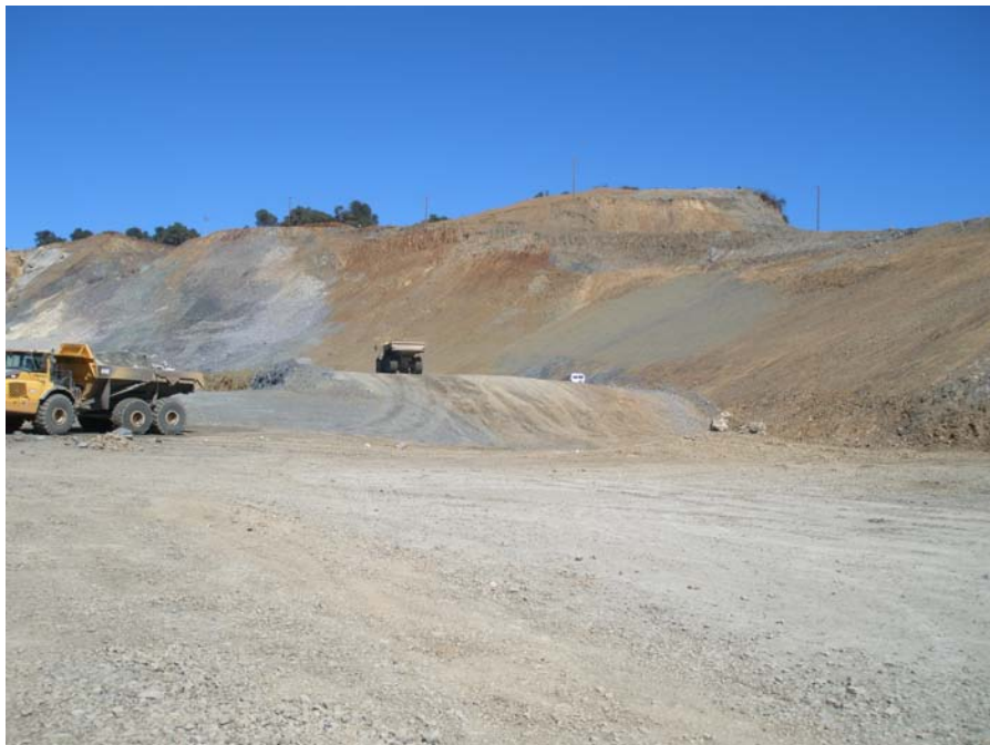
Photo 2: Upper portion of eastern highwall of North Quarry with slopes at final grade. First bench being cut to elevation at right side of photo. Dated September 26, 2013.
