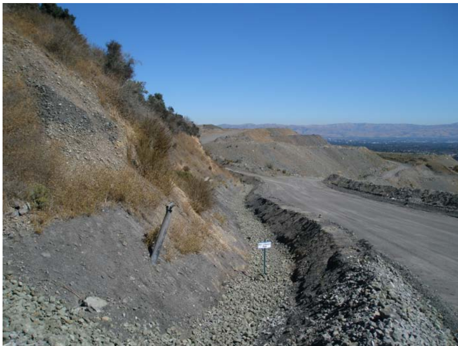
Photo 16: Western perimeter drainage ditch in EMSA. Ditch cleaned out and greenstone rock placed in bottom, looking northeast. Dated September 26, 2013.
