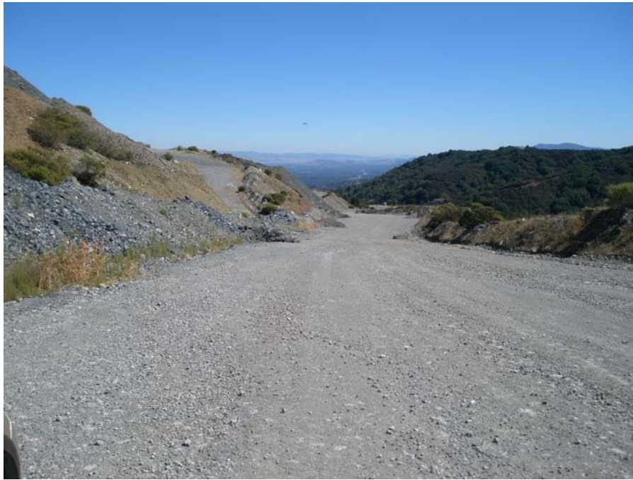
Photo 3: Check dams on WMSA haul road that were replaced with non-limestone materials, looking eastward. Dated September 26, 2013.
