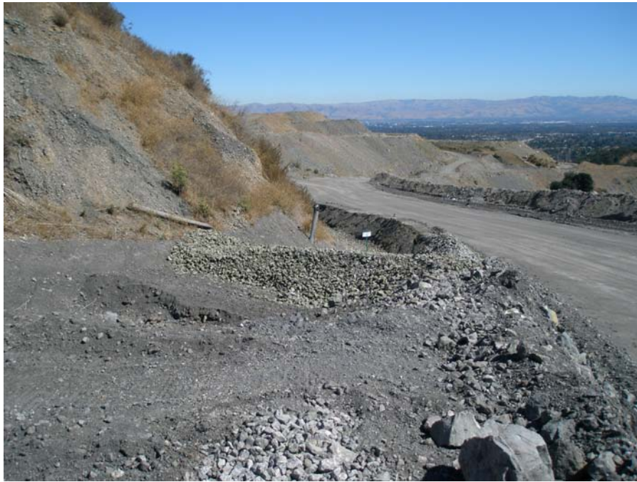
Photo 15: Sediment catch basin, greenstone rock weir and western perimeter drainage ditch in EMSA, looking northeast. Dated September 26, 2013.
