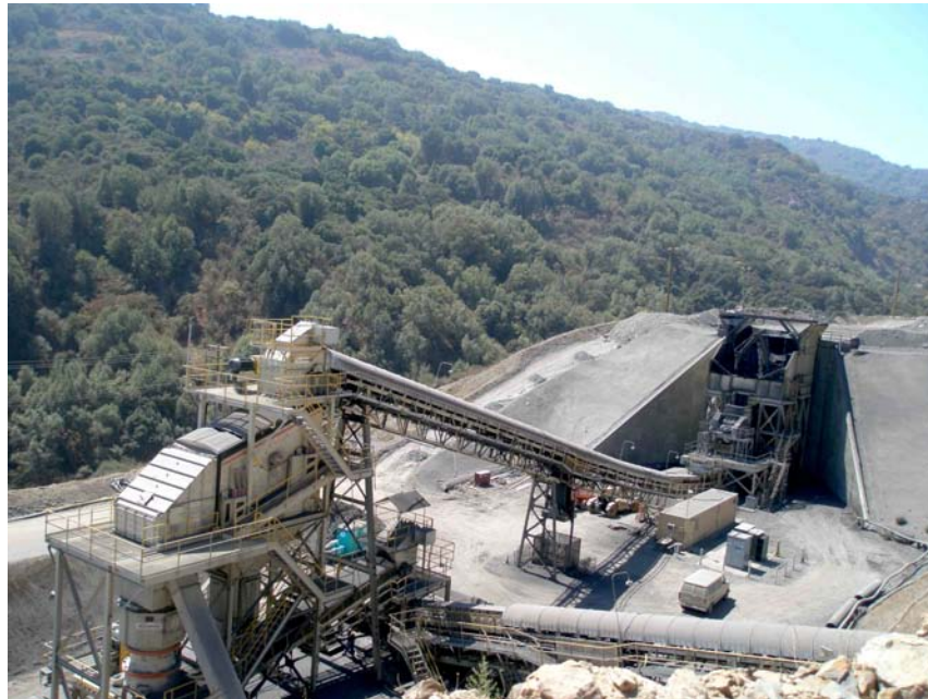
Photo 19: New primary and secondary crusher structures, looking southwest. Drainage from area will be collected and pumped into North Quarry for treatment before discharge. Dated September 4, 2014.
