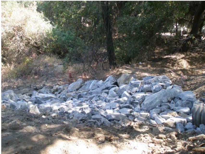
Photo 18: Pond 30 outfall to Permanente Creek, relined with coarser greenstone. Dated September 4, 2014.
