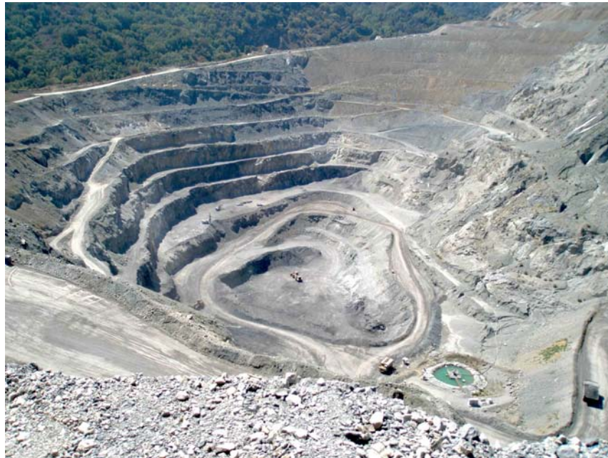
Photo 1: North Quarry, southwest portion. Waste rock material being placed at toe of western slope. Potential "Haul Road Slide" in eastern slope of WMSA, right of image. Floor elevation of quarry at approximately 650 feet msl. Dated September 4, 2014.
