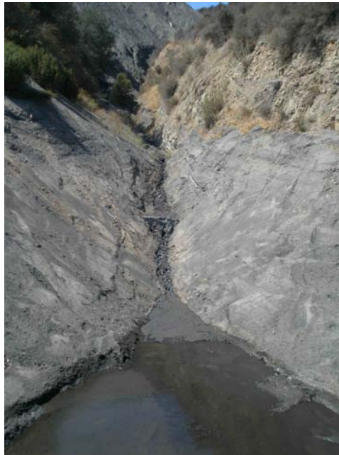
Photo 15: Sediment catch basin at toe of slope failure north of eastern end of 500-foot long conveyor tunnel in Crusher/Support Area, looking west. Dated September 4, 2014.
