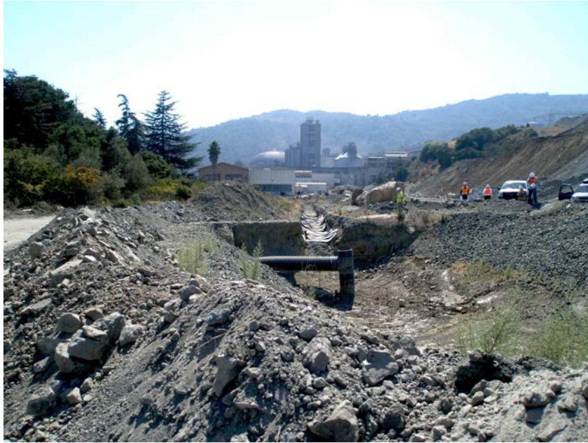
Photo 17: Pond 30 lowest pond in EMSA and drains into Permanente Creek, looking south at cement plant. Walls of pond and drainage ditch relined with greenstone. Dated September 4, 2014.
