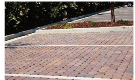
Pervious pavement area
