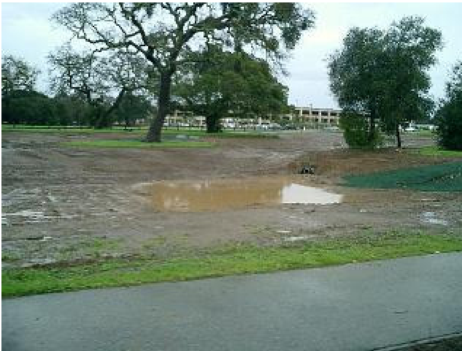
Storm Water Detention Basin (note: revegetation has not yet been established in this photo)
