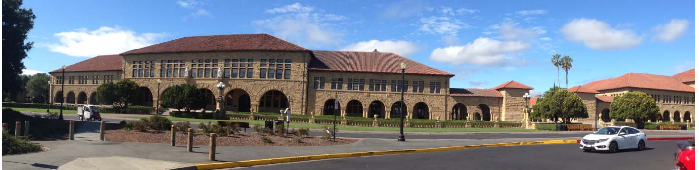
North east façade, 2016
