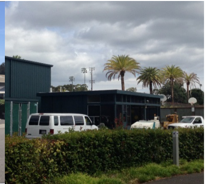
Name: 09-160 Auxilliary Shops Bldg. Original Date: 1962 Architect: Unknown
