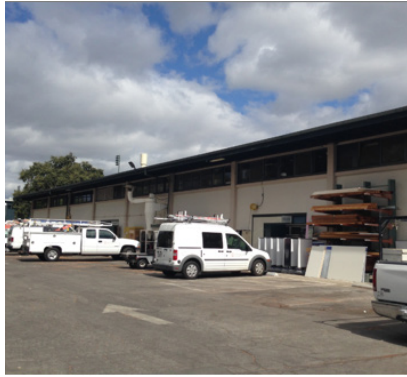
Name: 09-100, 315 Bonair Siding Original Date: 1961 Architect: Clark, Stromquist, Potter & Ehrlich
