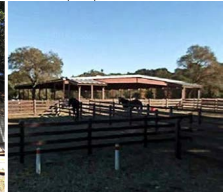
Name: 14-850, Riding Ring Original Date: 1958 Architect: Spencer & Lee
