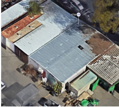
Name: 09-176, Operations & Maintenance Original Date: 1966 Architect: Unknown
