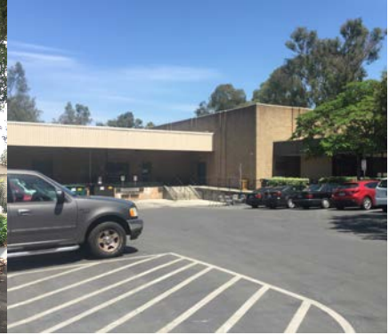
Name: 09-410, Stanford Auxiliary Library Original Date: 1973, addition (1992) Architect: Unknown (1969), David T. Takamoto (1992)
