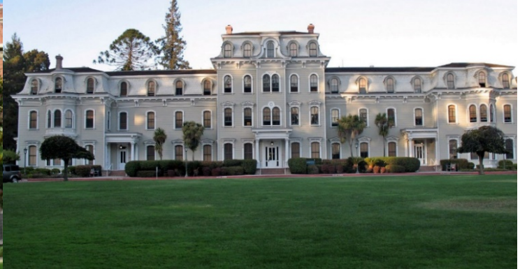
Mills Hall, Mill College (1871)
