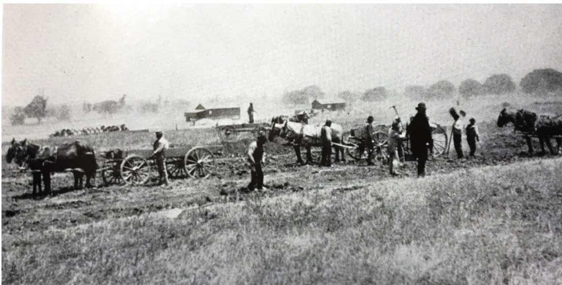
Clearing the land to begin construction of the Inner Quadrangle
