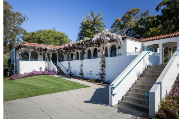
Vera M. Long Building, Mills College (1930)
