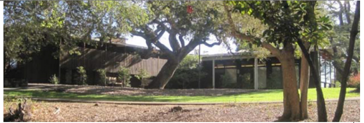
View of main building from west facade, 2014
