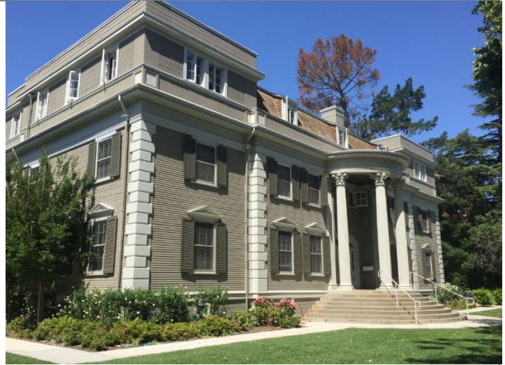
View of southeast corner, 2016
