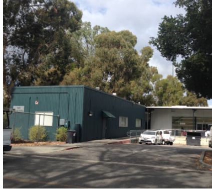
Name: 09-110, 340 Bonair Siding Original Date: 1962, addition 1971, addition 1973, addition 1979, addition 1985 Architect: Robert E. Jones structural engineer (1962), R. A. Rotondo structural engineer (1971), Office of Planning (1973), Vanderson Construction Inc. (1979, 1985)
