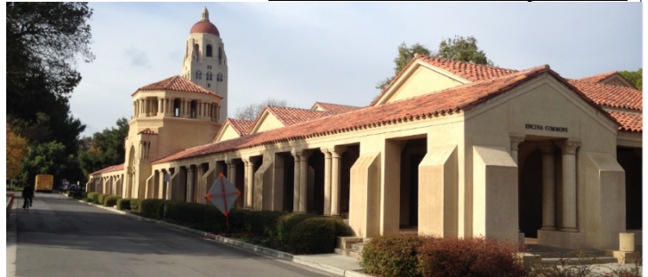
View of Encina Commons south façade, 2016
