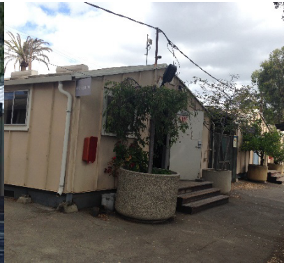
Name: 09-173T, Irrigation & Break Room Original Date: 1961 Architect: Lawrence G. Brian
