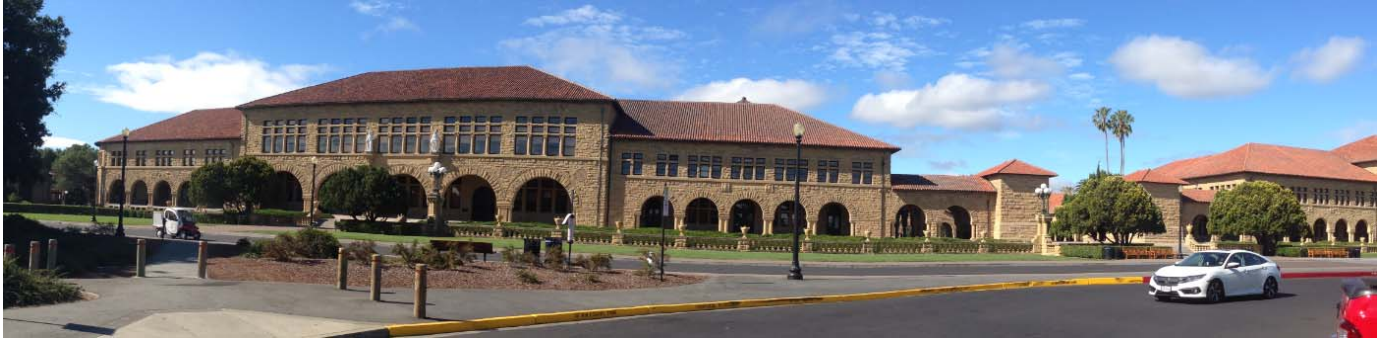
North east façade, 2016
