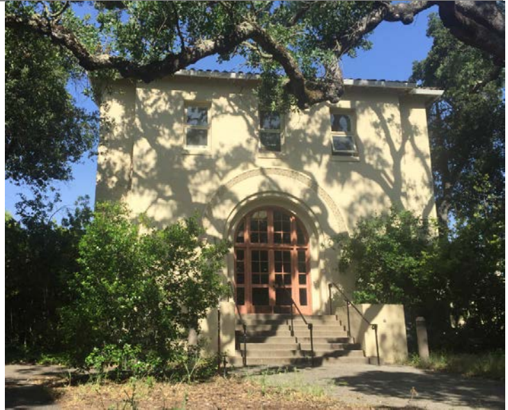
View of east façade, 2016
