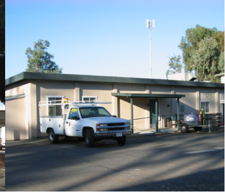
Name: 09-130, Steam Fitters Shop Original Date: 1965 Architect: Spencer, Lee & Busse
