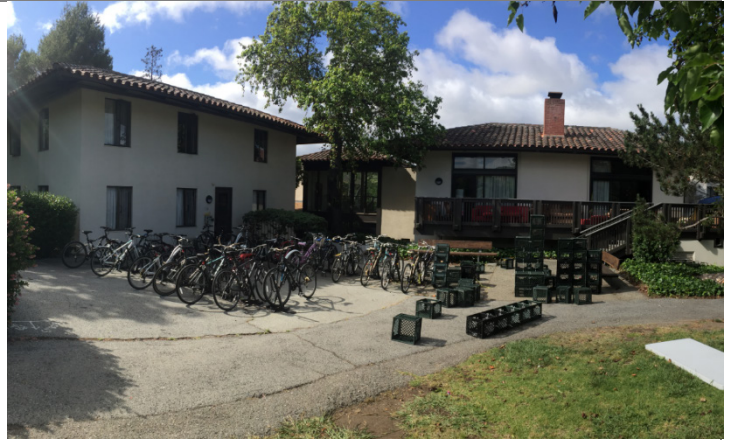
View of east façade, 2016
