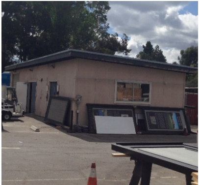
Name: 09-135, Carpenter Shop Storage Original Date: 1962 Architect: Unknown
