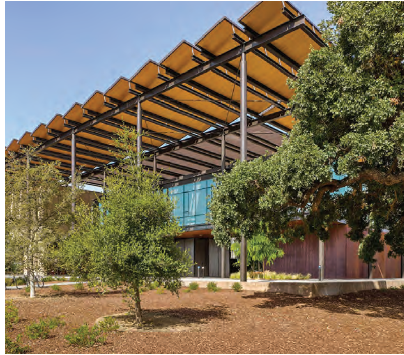
Central Energy Facility
