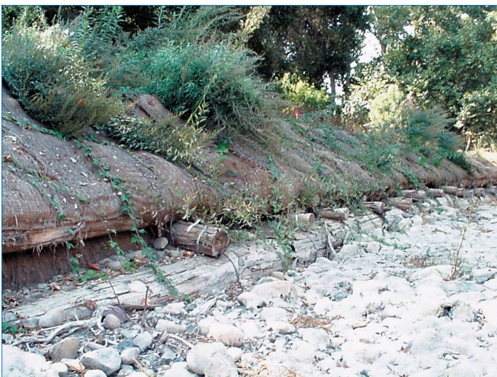
Biotechnical erosion repair.
